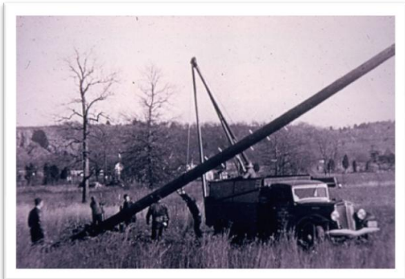
SETTING ONE OF FIVE '65 MASTS
